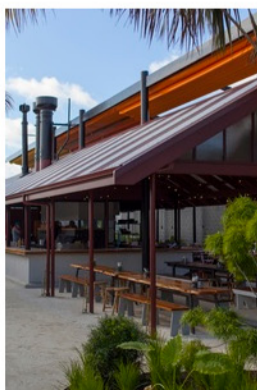
Striped corrugated iron was used for the roof.
